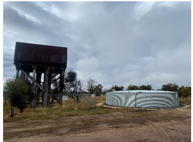
Water tank at Kylie Siding
