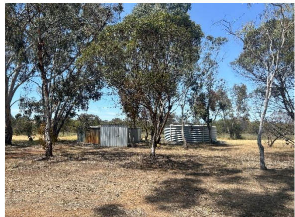
Tanks and pump house
