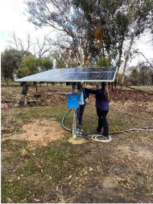
Solar panel and pump
