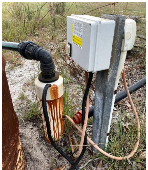
Rees Road bore pump setup
