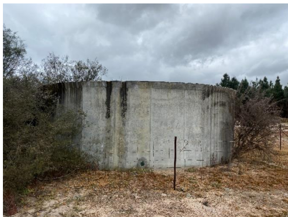
Tank at Gorn Road
