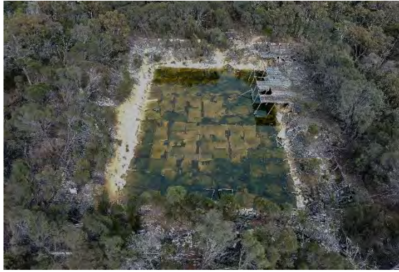
Plate 5. View north of Hillman Dam with collapsed asbestos roof visible in the water (source: Frank Chia for Shire of West Arthur)
