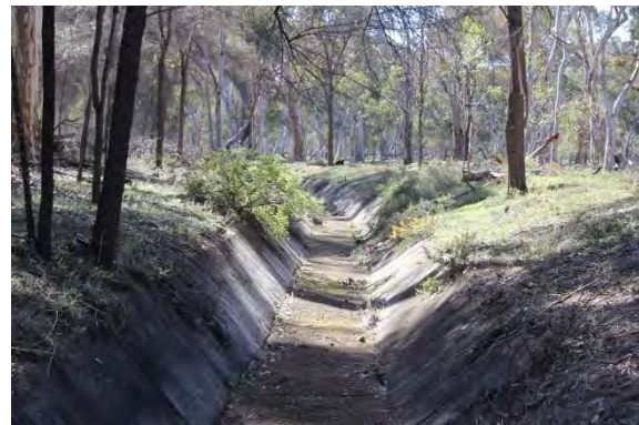
Plate 4. Stone channels that feed water from Julikan Rock catchment into Hillman Dam (source: LocationsHub)
