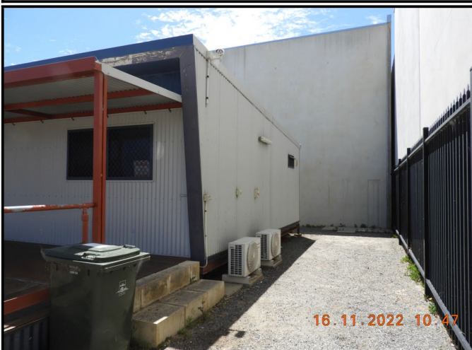
Photo 5 : Quick Over view:- South front Corner – all exterior lining is in corrugated colour-bond sheeting
