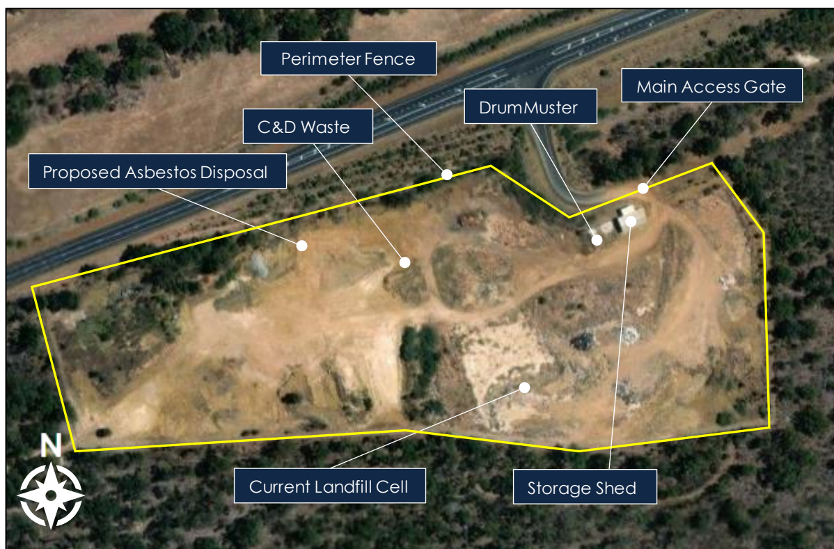
Figure 1.2 - Facility layout (Aerial Image from Nearmap October 2022)
