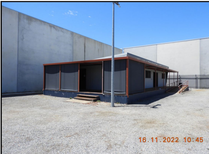
Photo 1 : NOTE - if there is no narration in the boxes under the photos, then there is nothing of structural significance to report or it's a repetitive issue. In conjunction the inspector may make comments, observations & highlight major or minor serviceability defects & maintenance issues
