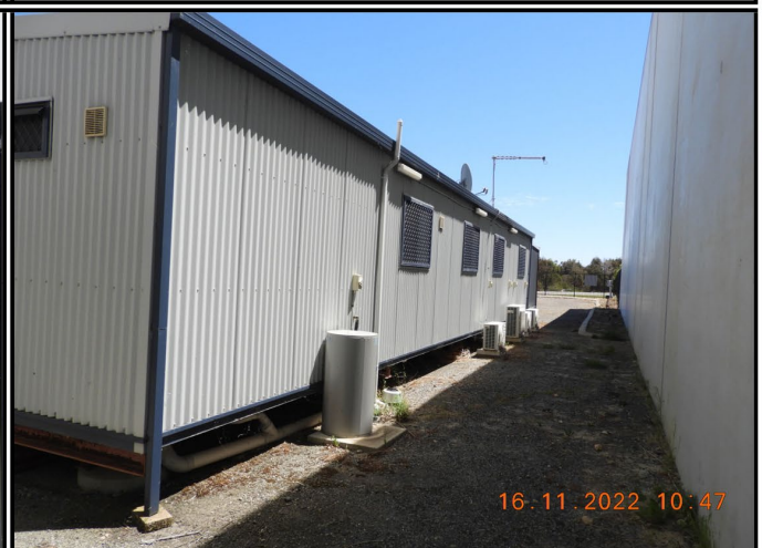
Photo 6 : East rear Corner
