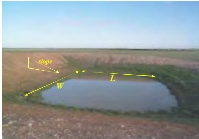
Figure D1: Measurements that should be taken when inspecting a farm dam (in addition to water depth)
